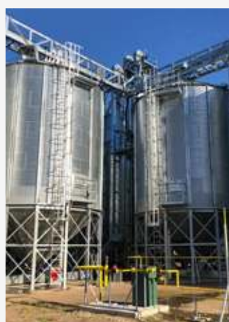
Country: Latvia Project: LIS Year: 2019 Continuous flow dryer GL7, 25 t/h (wheat) Chain conveyor K100, 60 t/h Drive-over intake pit PB3.5x10m Flight conveyor S80L with bend, 80 t/h x 3 Chain conveyor K100, 80t/h Flight conveyor S80L with bend, 60 t/h Bucket elevator E80, 60 t/h Chain conveyor K100, 80t/h Chain conveyor K100, 100 t/h.
