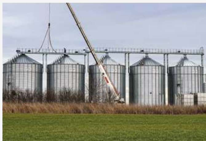
Country: Romania Year: 2020 Chain conveyor K100, 80t/h x 8 Bucket elevator E80, 80t/h x 6 Two-way dividers, three-way dividers, grain brakes, electrical slides, manual slides Conveyor supports.
