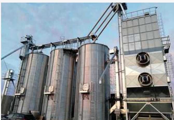
Country: Estonia Year: 2018 Bucket elevator E80, 80 t/h x 2 Batch dryer BXL76 Chain conveyor K100, 100 t/h.
