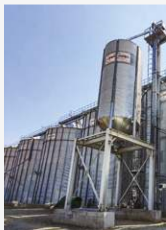
Country: Romania Year: 2020 Chain conveyor K100, 80t/h x 8 Bucket elevator E80, 80t/h x 6 Two-way dividers, three-way dividers, grain brakes, electrical slides, manual slides Conveyor supports.
