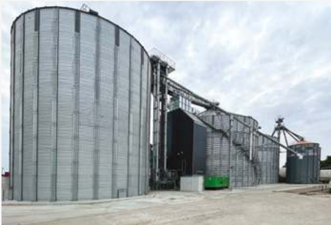
Country: Germany Year: 2023 Chain conveyor K120, 120t/h Flight conveyor S150, 120t/h Bucket elevator E150, 120 t/h Chain conveyor K40, 30t/h Continuous grain dryer GL10 3-way and 2-way valves.
