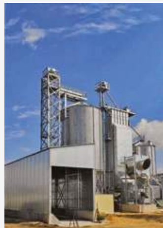
Country: Russia Year: 2020 Chain conveyor K120, 100t/h x4 Bucket elevator E80, 100t/h x 3 Flight conveyor S100, 100t/h Accessories Continuous Flow Dryer GXL11, 60 t/h (wheat).
