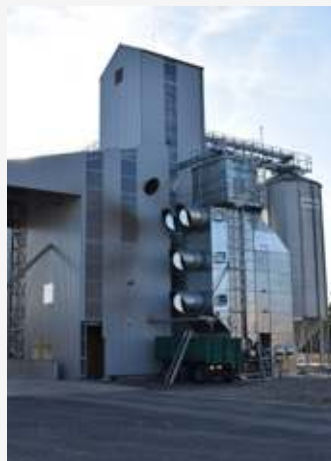
Country: Latvia Project: farm Siecini Year: 2017 Continuous flow dryer GL6, 21 t/h (wheat) Chain conveyors K100, 100 t/h Bucket elevators E80, 80 t/h.
